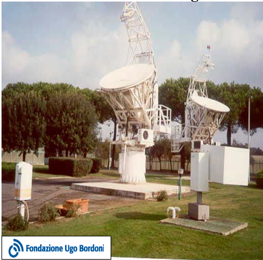
ITALSAT beacon receiving station
